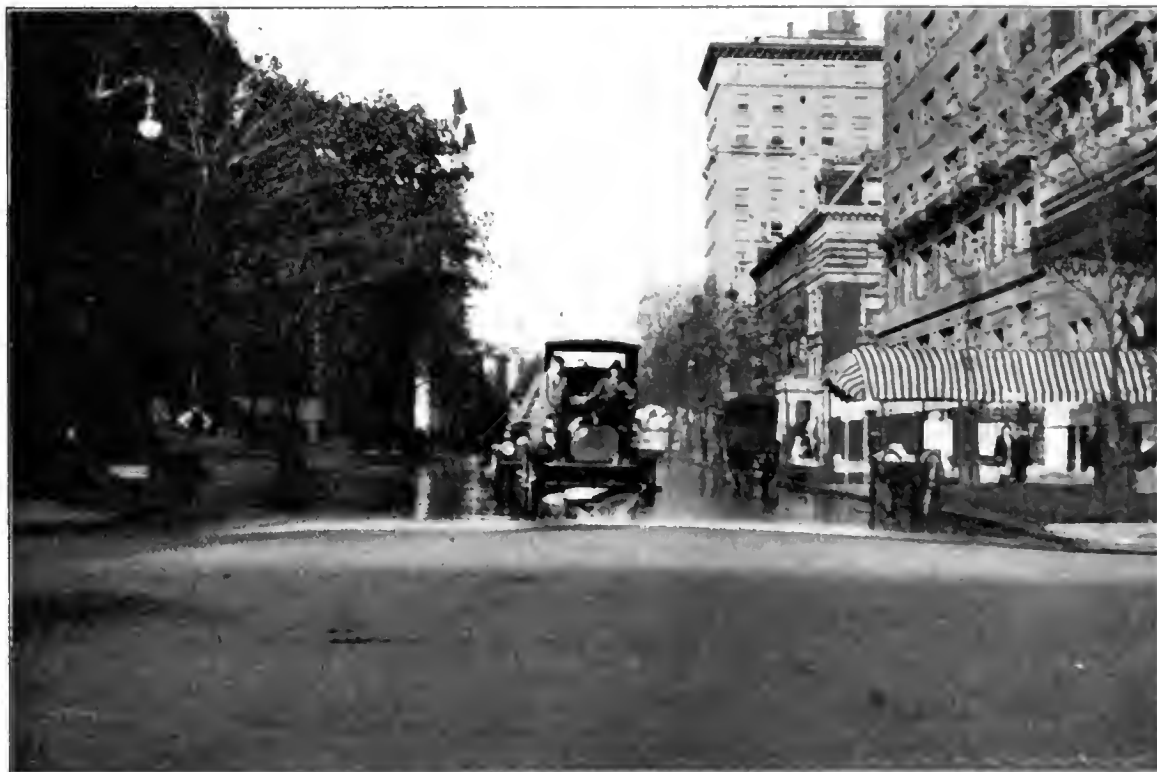
Motor-driven power flusher Flushes entire width of street.
